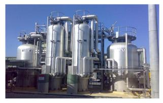
Fig 5 Picture of CambiTHP<sup>TM</sup> in WWTP Brisbane
